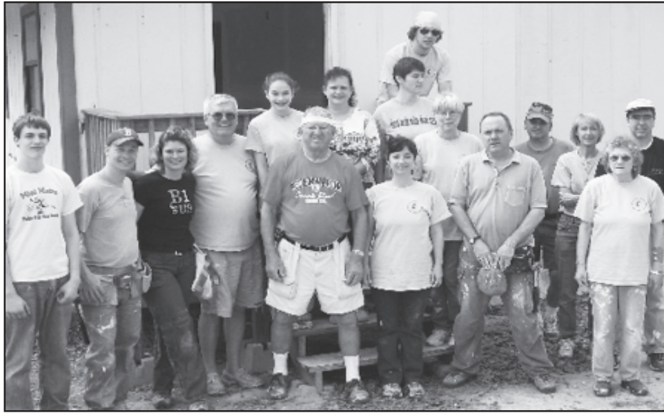
Fifteen Vermont volunteers including ten members of the Covenant Community Church of Jericho Road took part in a mission trip to Gulfport, Mississippi to repair Katrina-damaged homes.
